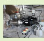
and supplied the stainless steel pump system to the Barbers Cattle Market in Shropshire. The washdown set (Hidroboost) features cost-effective intelligent variable speed drives which optimise system efficiency with a duty/assist configuration to compensate for the varied demand of the market. After reviewing the original systems' location within a 4 metre deep chamber, T-T designed the booster set to be surface mounted for ease of access, service and maintenance.
